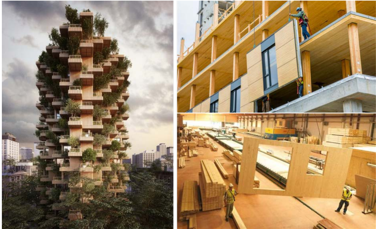
Figure 41. Mass timber, prefab assembly
